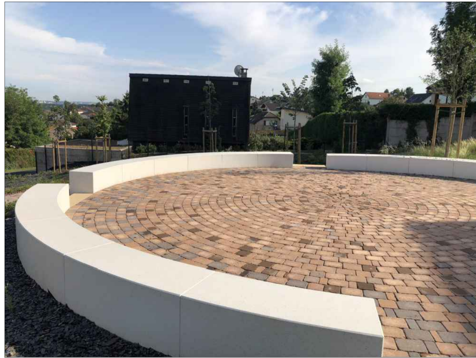
CIRCULAR BENCH FOR PLAY AREA Around the play area Concrete Length : 2500mm; Width: 500mm; Height: 500mm
